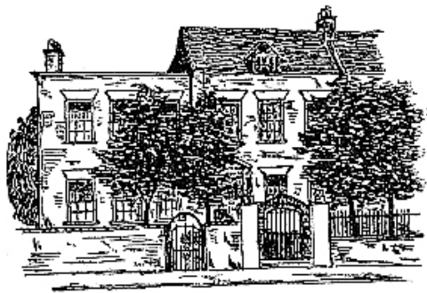
SKETCH OF 29 STEPNEY GREEN MADE BY P. B. IN 1920. THIS SHOWS THE PROPERTY AS ACQUIRED BY ROLAND PHILIPPS WITH THE OLD SIDE ENTRANCE GATE
